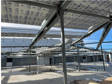
Beginning of installation
