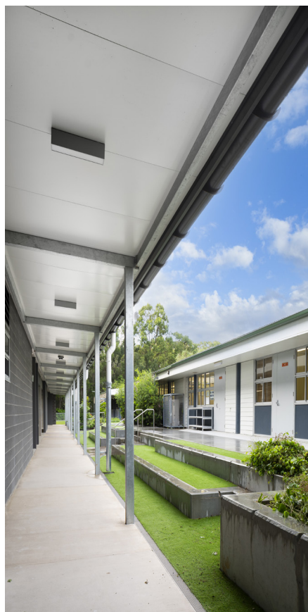
Underside of External Connecting Walkway
