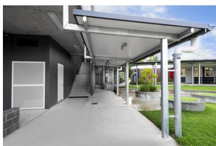
External Connecting Walkway with HDG Structural Steel
