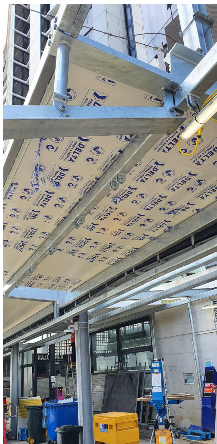
Delta DualCore being installed
