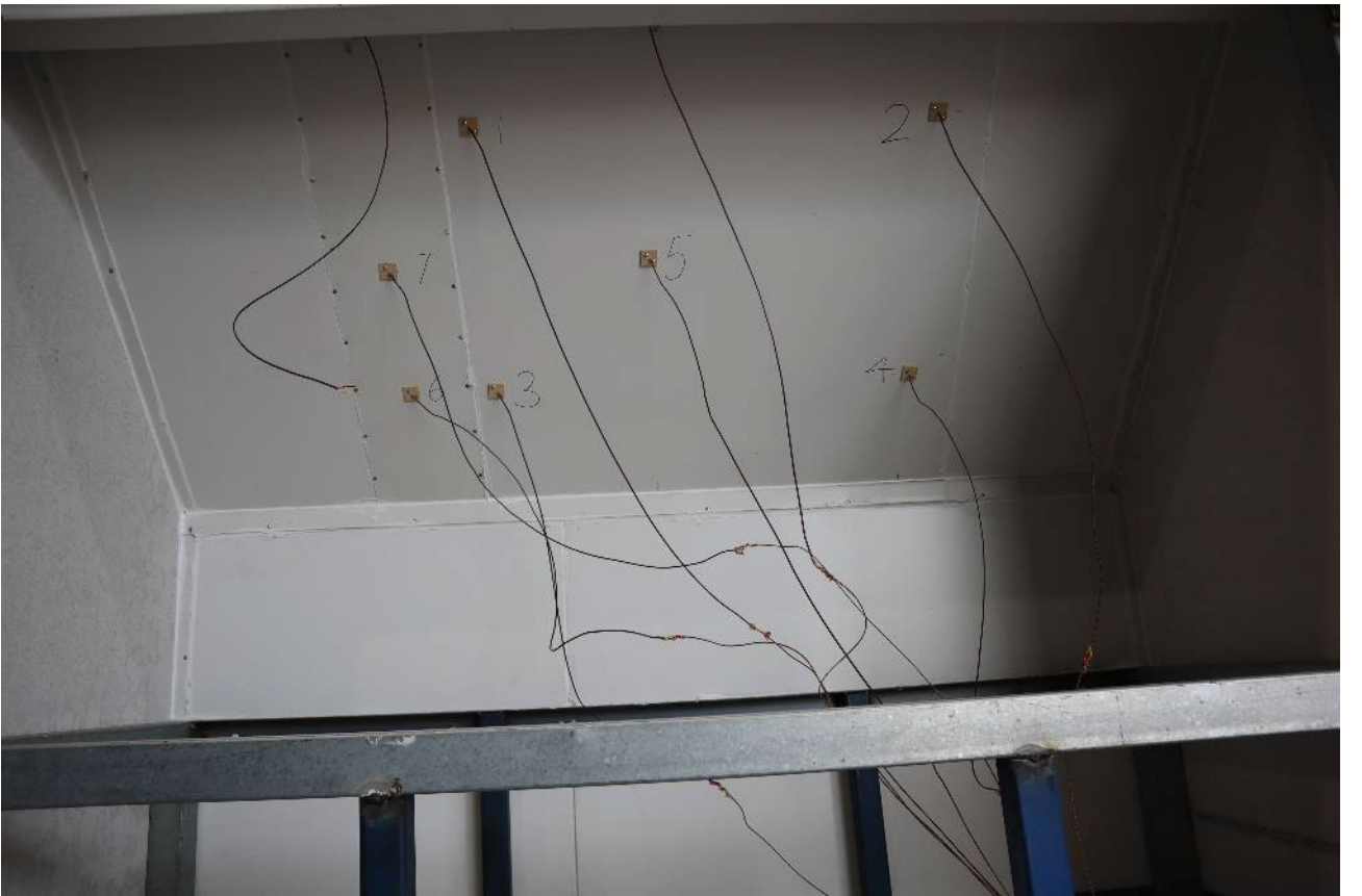
PHOTOGRAPH 18 – UNEXPOSED FACE OF THE ROOF CAVITY AFTER THE CONCLUSION OF TESTING
