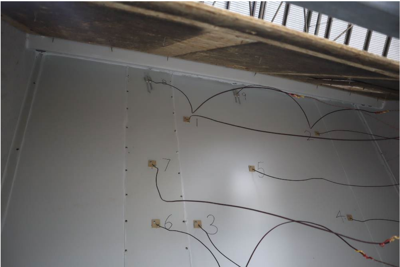
PHOTOGRAPH 3 – INSTRUMENTATION OF THE ROOF CAVITY
