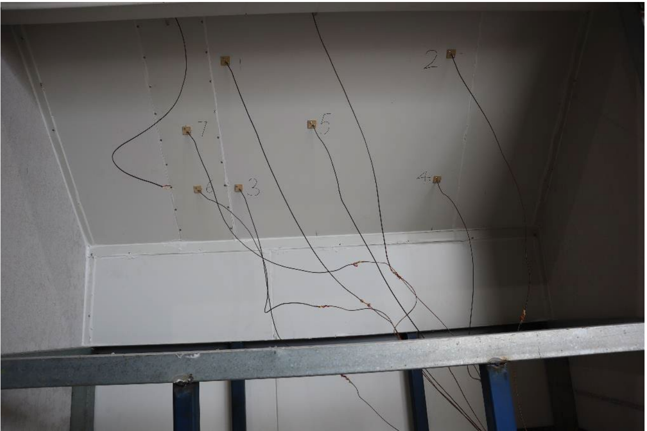
PHOTOGRAPH 17 – UNEXPOSED FACE OF THE ROOF CAVITY AFTER THE CONCLUSION OF TESTING
