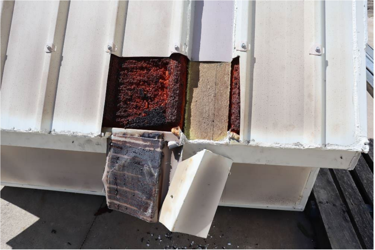
PHOTOGRAPH 19 – UNEXPOSED FACE OF THE ROOF CAVITY AFTER THE CONCLUSION OF TESTING
