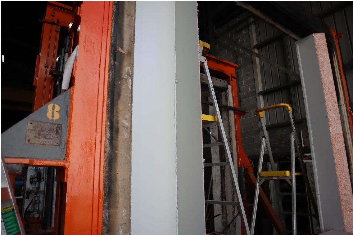
PHOTOGRAPH 1 – CONSTRUCTION OF SPECIMEN – FORMING UP OF THE TWO REBATE CORNERS
