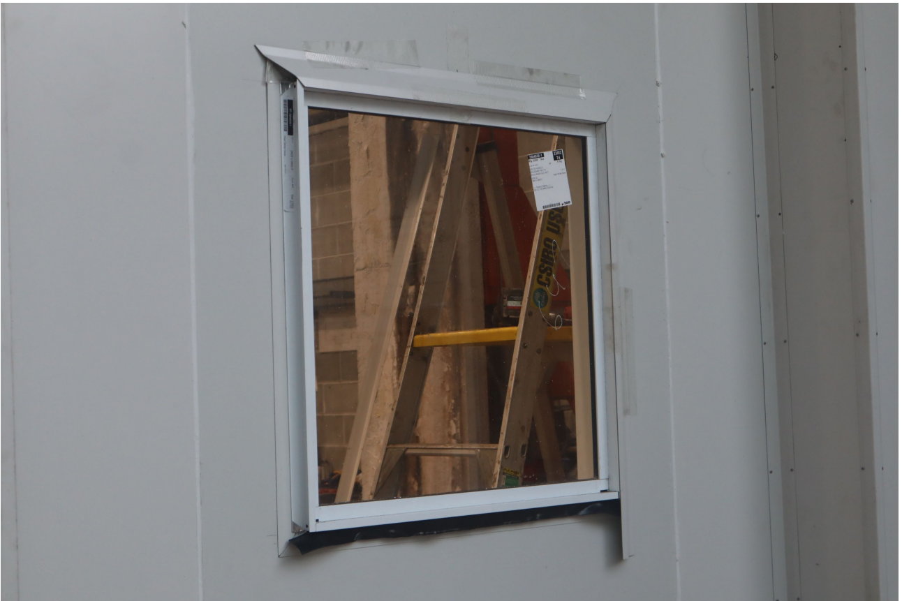
PHOTOGRAPH 3 – CONSTRUCTION OF SPECIMEN – INSTALLATION OF THE WINDOW FLASHING
