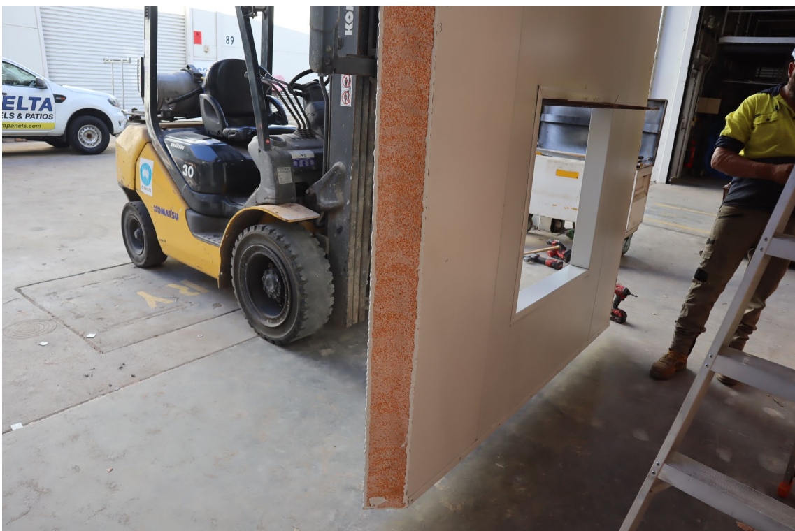
PHOTOGRAPH 2 – CONSTRUCTION OF SPECIMEN – INSTALLATION OF THE MAIN WALL SECTION
