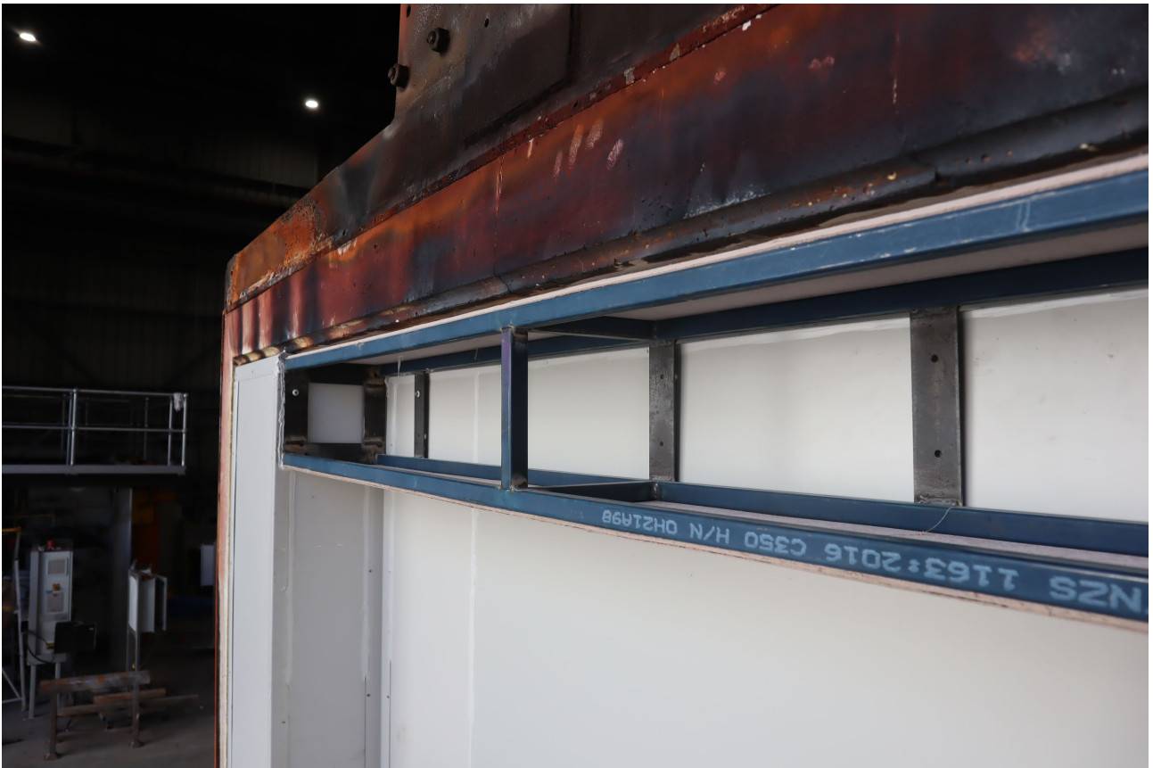
PHOTOGRAPH 5 – CONSTRUCTION OF SPECIMEN – EAVES DETAIL
