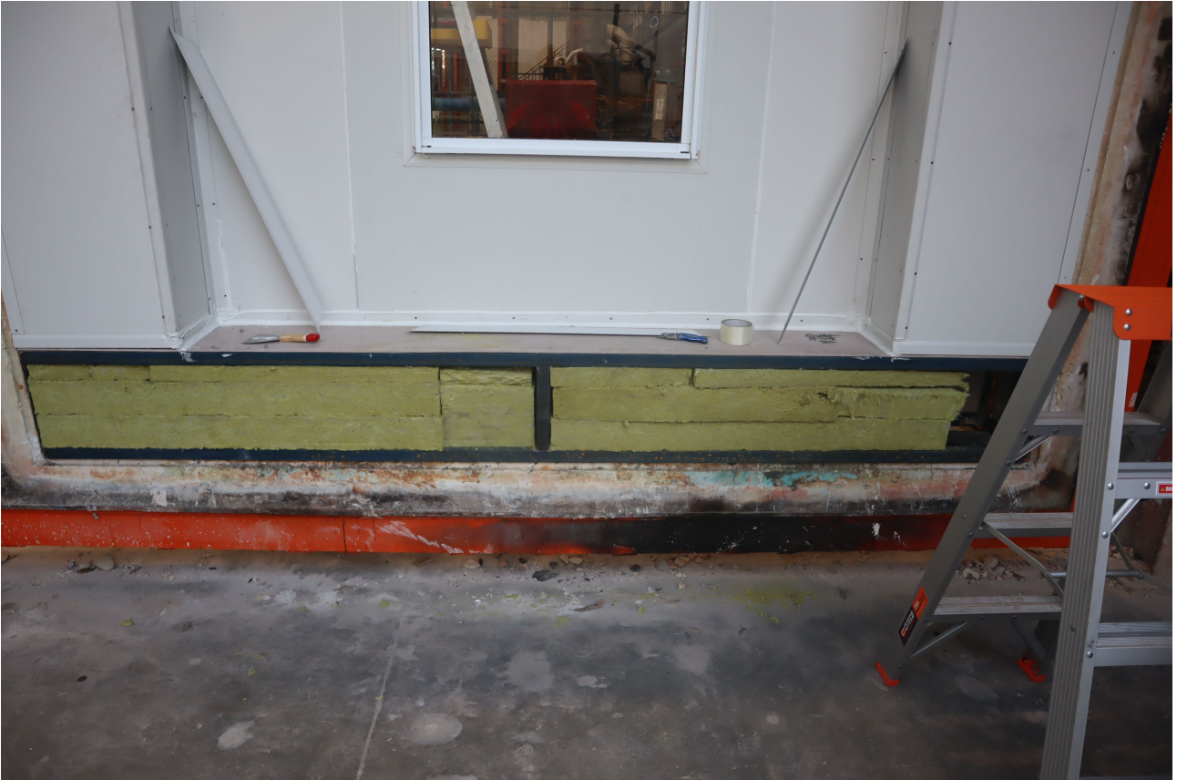
PHOTOGRAPH 4 – CONSTRUCTION OF SPECIMEN – SILL DETAIL
